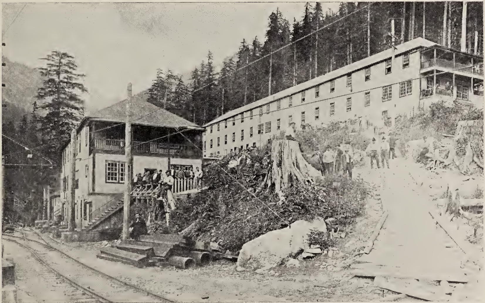
BUNK-HOUSE AND DINING-HALL, MODERN EQUIPMENT, AT B.C. MINE CAMP.
